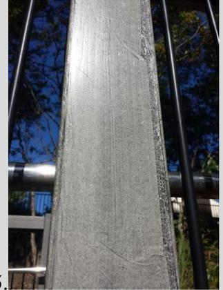
Photo 6 below showing where deterioration has exposed glass fibres.
