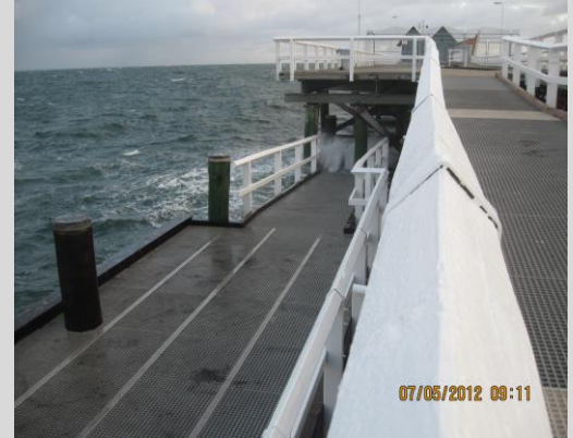
EnviroGrate H50 Heavy Duty 38x38 grid with 11mm thick load bars & 27x27 openings to withstand strong ocean surge, BUSSELTON
